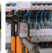
Measurement of phase sequence.
